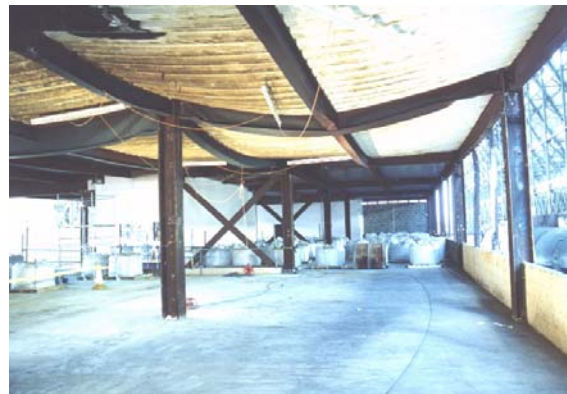
Figure 5-1 Restrained structural steel framing sustained large deflections without collapse during a fire test in Cardington, UK - CORUS Steel
