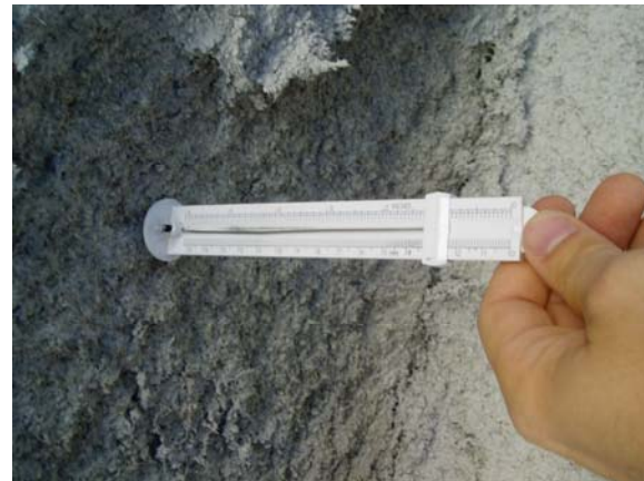
Figure 7-5 thickness testing of SFRM – DeStefano & Chamberlain
