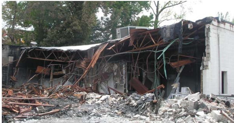
Figure 7-10 Fire damaged steel joists - DeStefano & Chamberlain
