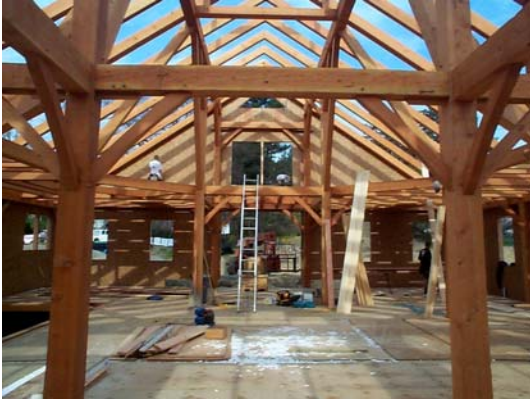
Figure 10-3 Timber frame structures exhibit good fire performance - DeStefano & Chamberlain
