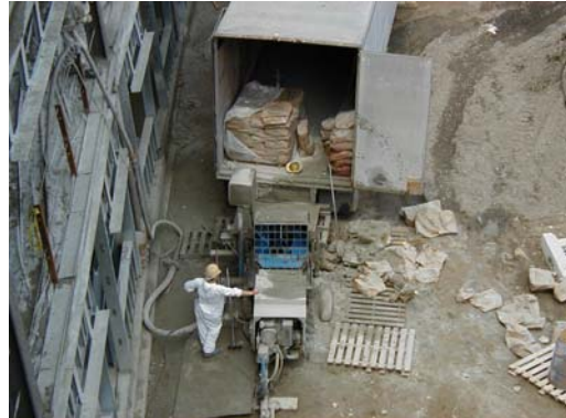
Figure 1-2 Spray fireproofing operation – DeStefano & Chamberlain
