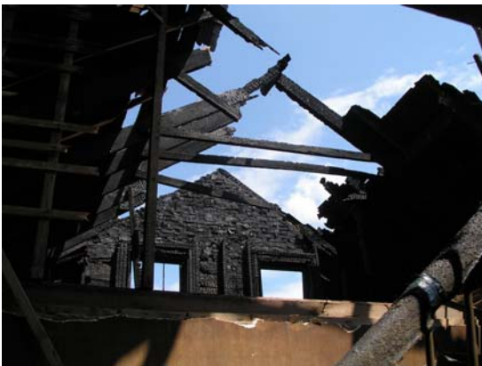
Figure 10-1 Fire damaged light wood framing - DeStefano & Chamberlain
