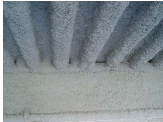
Figure 7-9 Flutes of metal deck have not been completely filled over beam – DeStefano & Chamberlain
