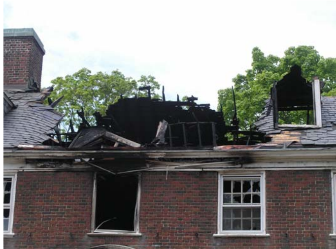
Figure 9-1 Masonry bearing walls sustained no significant damage in fire - DeStefano & Chamberlain
