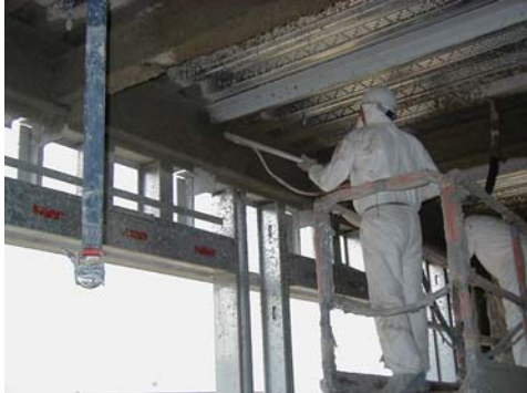
Figure 7-1 Application of SFRM – DeStefano & Chamberlain
