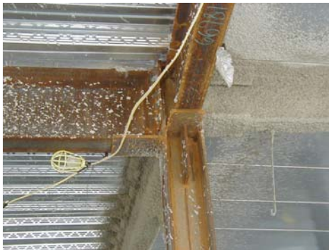
Figure 7-3 SFRM applied over bare steel – DeStefano & Chamberlain
