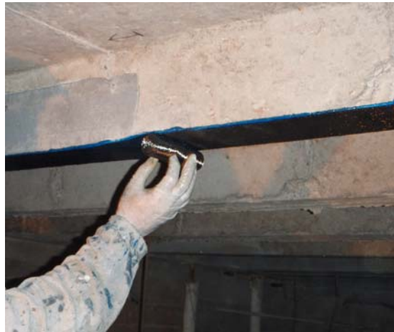
Figure 8-3 FRP unidirectional strengthening of concrete joists - Degenkolb
