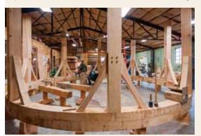
**Getting underway.** Some prefitting work was done with the structure upside down, which made working on the rotunda of this building more comfortable.
