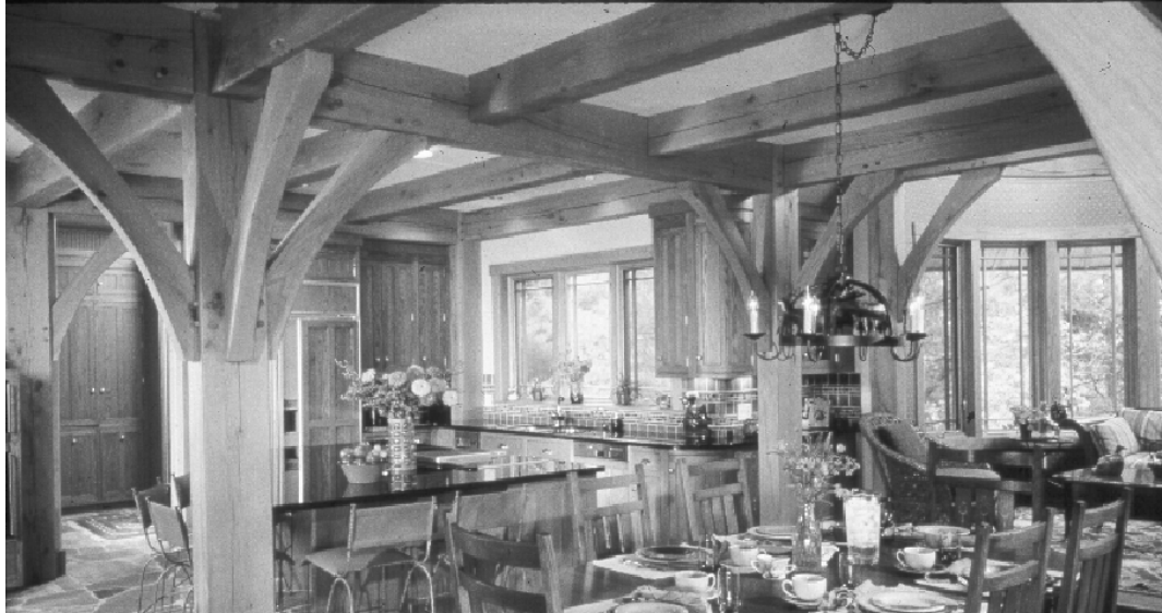
Figure 1-1 Typical Timber Frame (courtesy of Riverbend Timber Framing)
