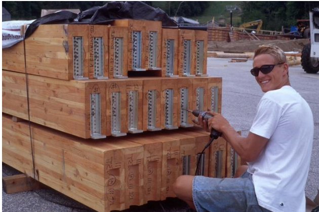
Figure 14 Pre-engineered galvanized steel connectors with a bearing seat and screws into the ends of the timbers
