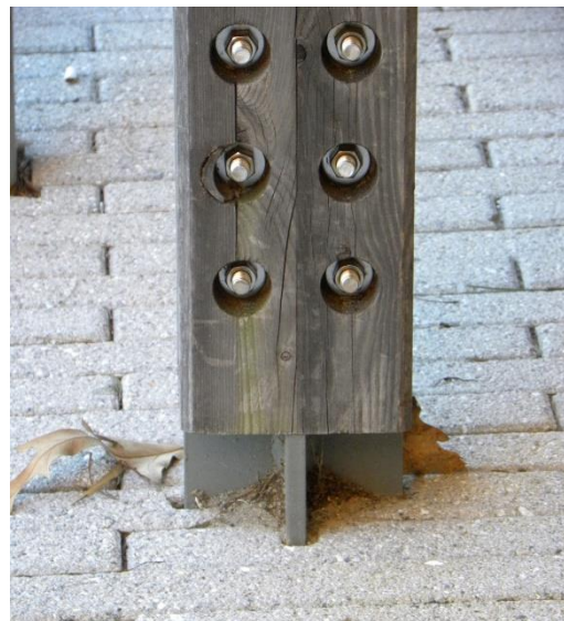
Figure 11 Elevated post base drains freely
