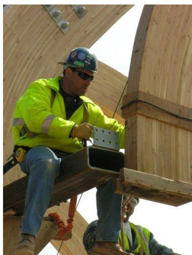
Figure 2 A glulam timber structure being erected by ironworkers
