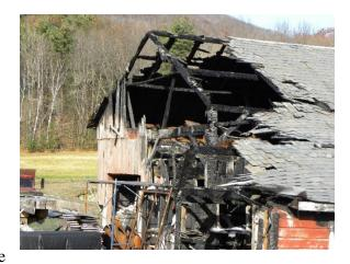
core of a timber from the heat of a fire, permitting the timber to continue to carry load.
