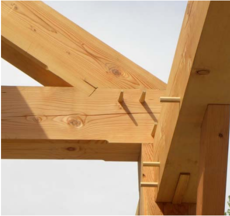
Figure 1 - Truss Heel Joint
